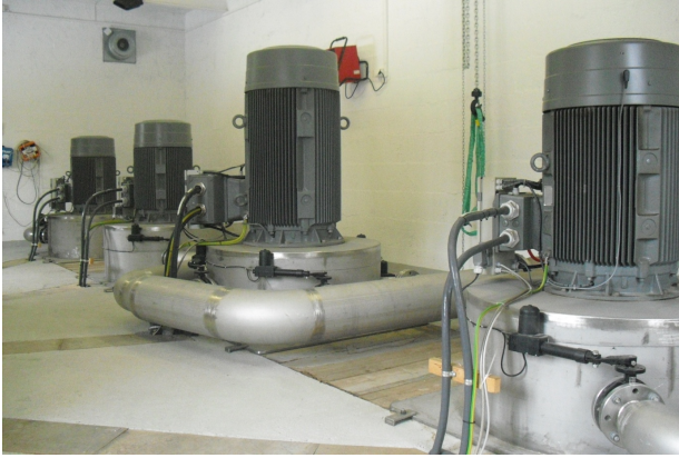
Figure 7: The four generator units in Sagbekken 2 and 3
