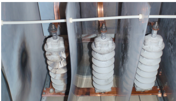
Figure 4: Broken surge arrester to the far-left
